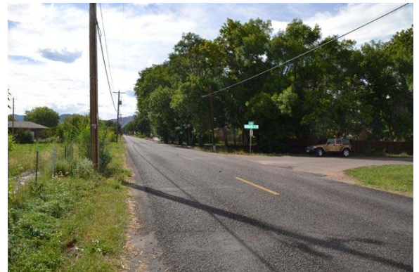
Paved Access/City Utilities
