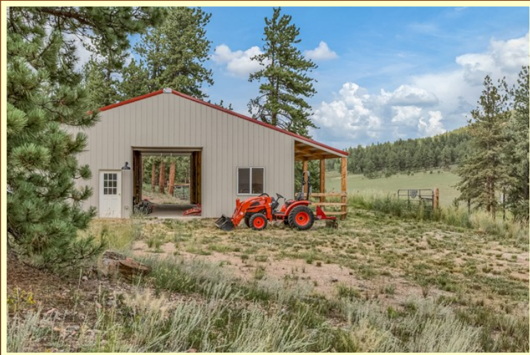
Pole Barn, Fenced, Cross-Fenced & Gated
